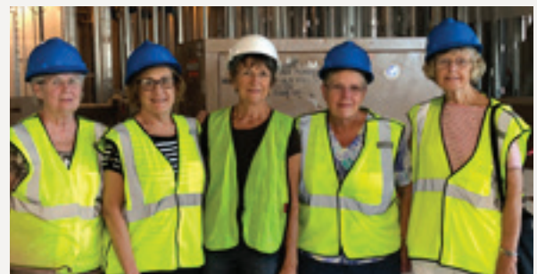
Some members of the Mercy Health Volunteer Board recently toured the new medical center construction site. Left to right: Pat Preston, Karen Driver, Alice Pasarela, Rita Rainwater and Connie Brantman.
