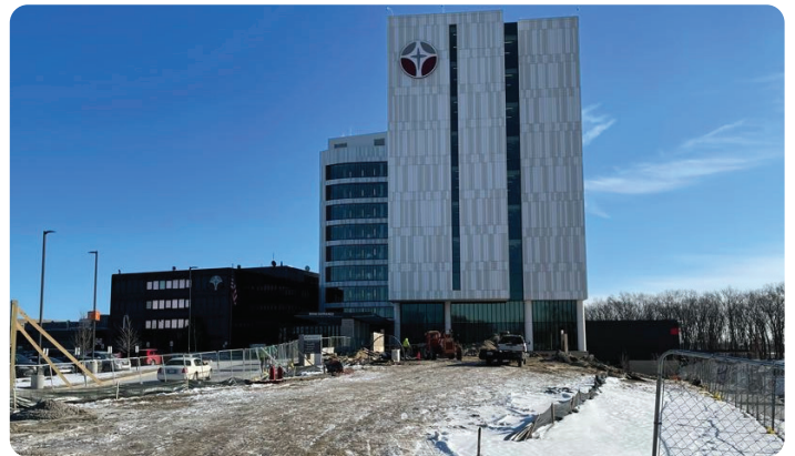
Current construction progress of the Healing Garden
