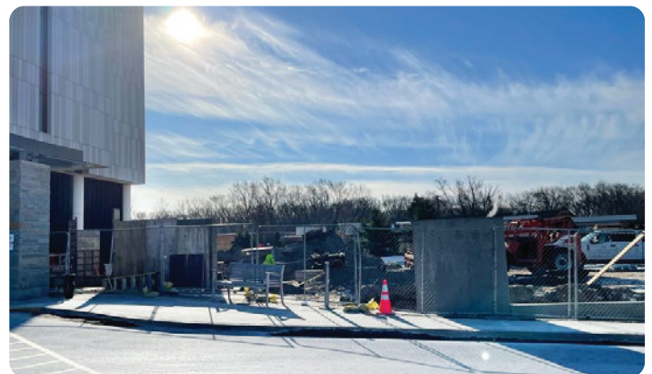
Current construction view of the entrance into the Healing Garden
